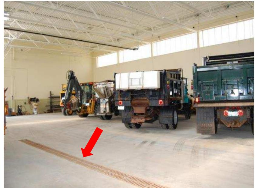
Any drips or spills from vehicles stored inside will be collected in a closed floor drain system preventing them from reaching the environment
