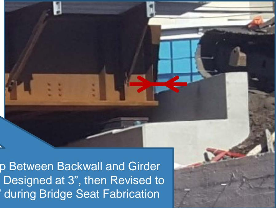
Gap Between Backwall and Girder End Designed at 3", then Revised to 10" during Bridge Seat Fabrication
